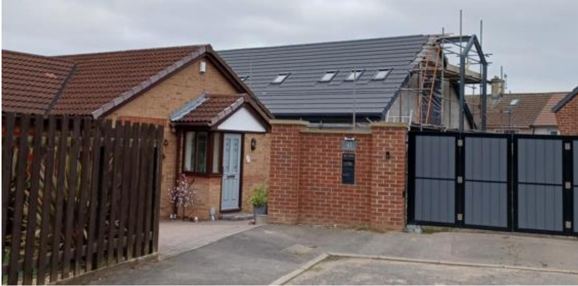
Figure 8: Photograph showing south elevation as built
