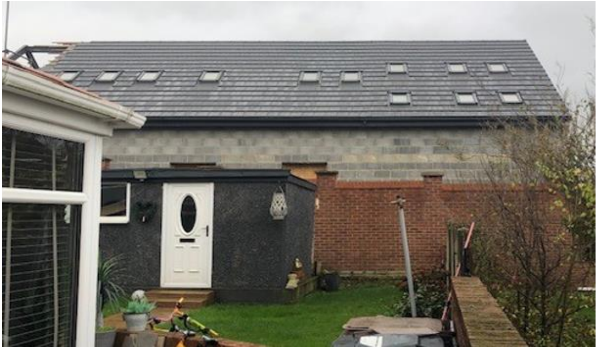
Figure 6: Photograph showing the north elevation as built.
